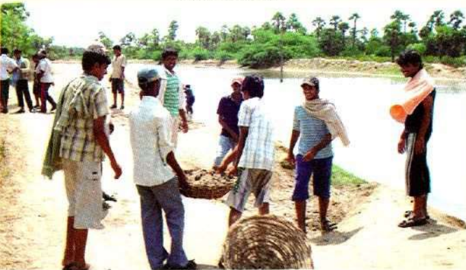
Strengthening the banks of the canals
