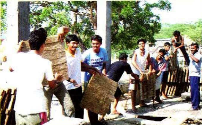
Helping hands at building houses for rural poor- camp at Lakshmiapuram
