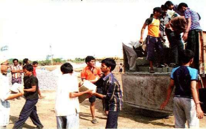
Village rebuilding activities at Talagadadeevi village, Nagayalanka
