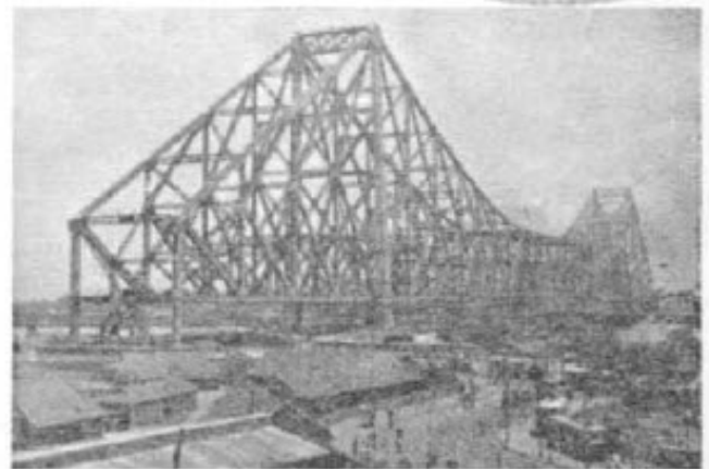
5. Howra Bridge - Calcutta.
