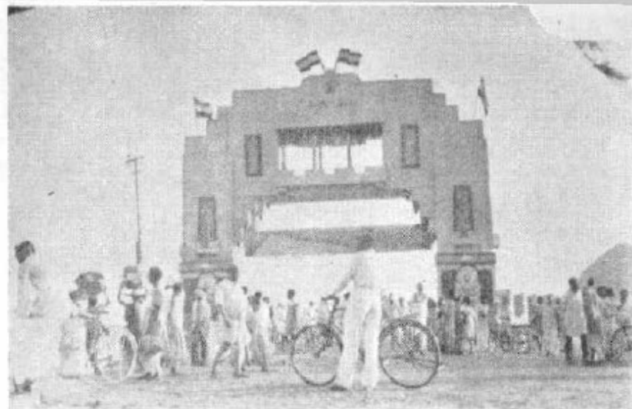
2. Entrance to New Bridge over the Krishna.
